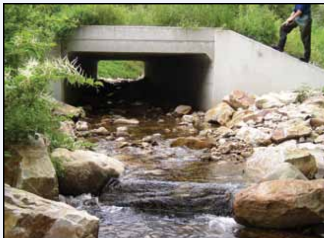
Looking upstream at the new concrete box culvert. Note the rock grade control weir constructed downstream of the project to maintain the streambed elevation at the outlet.
