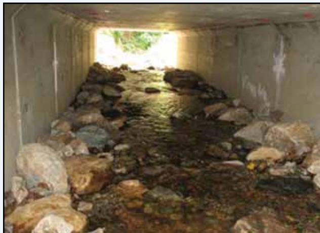
Stream substrate within the culvert was constructed to mimic natural stream conditions and withstand the forces of high flows.
