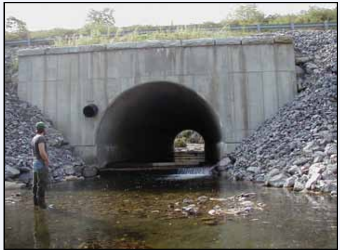
Broad Brook culvert with outlet perch.
