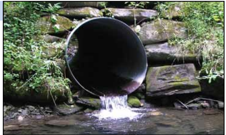
Perched outlet, scour pool and bank erosion.
