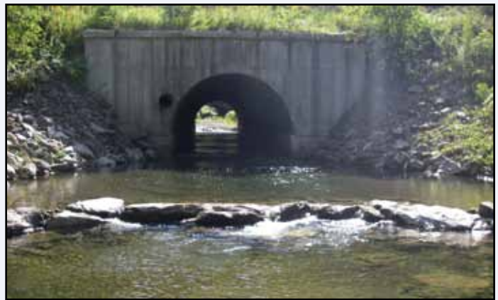
Constructed rock weir eliminates outlet perch.
